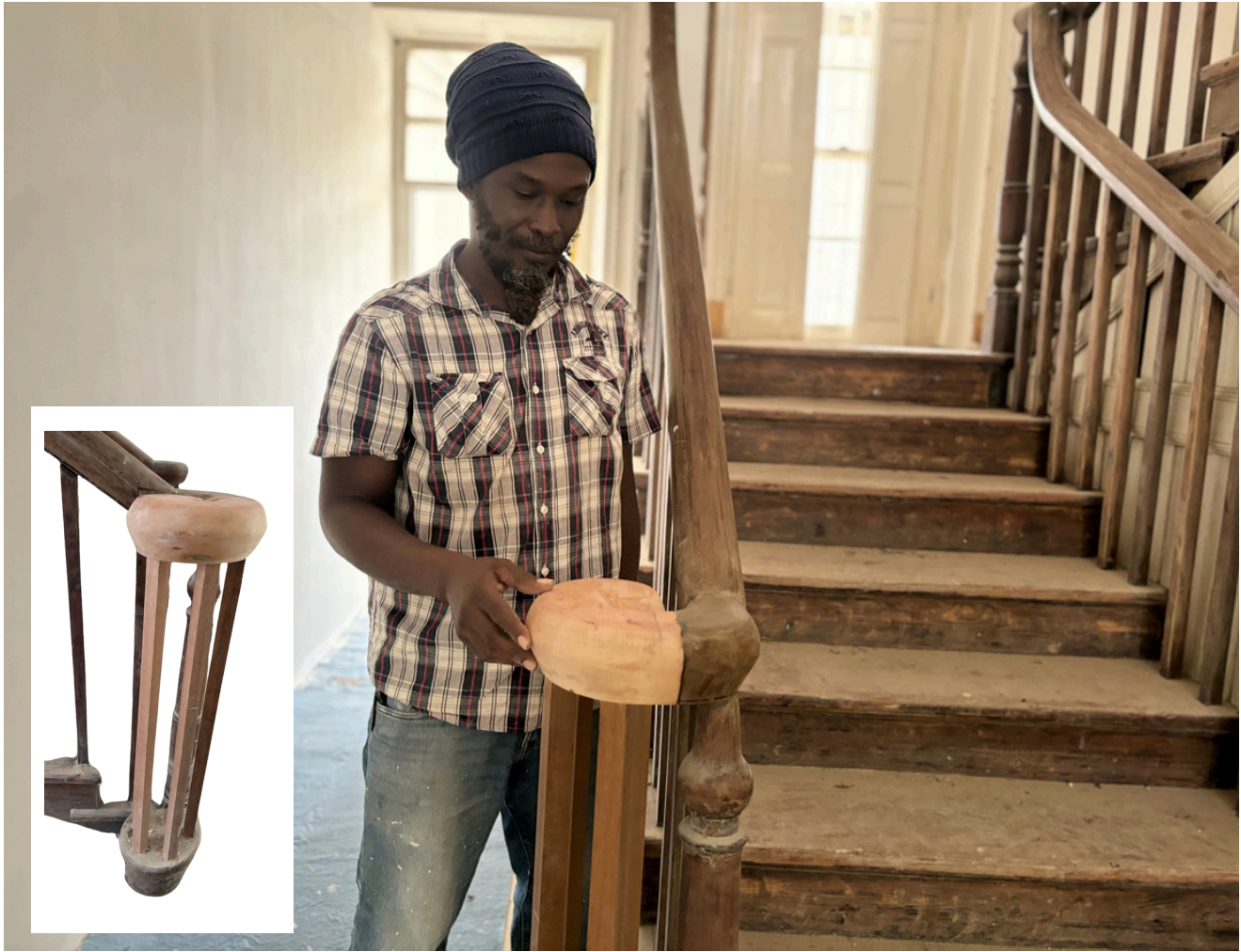
Junior Sealy examining his work on the curved newel post, a full view is inset.
