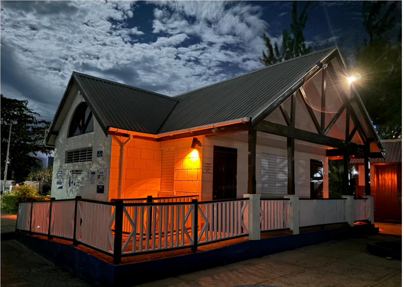
One of the turtle-friendly amber LED lights that was installed at the Pebbles Beach Facility.
