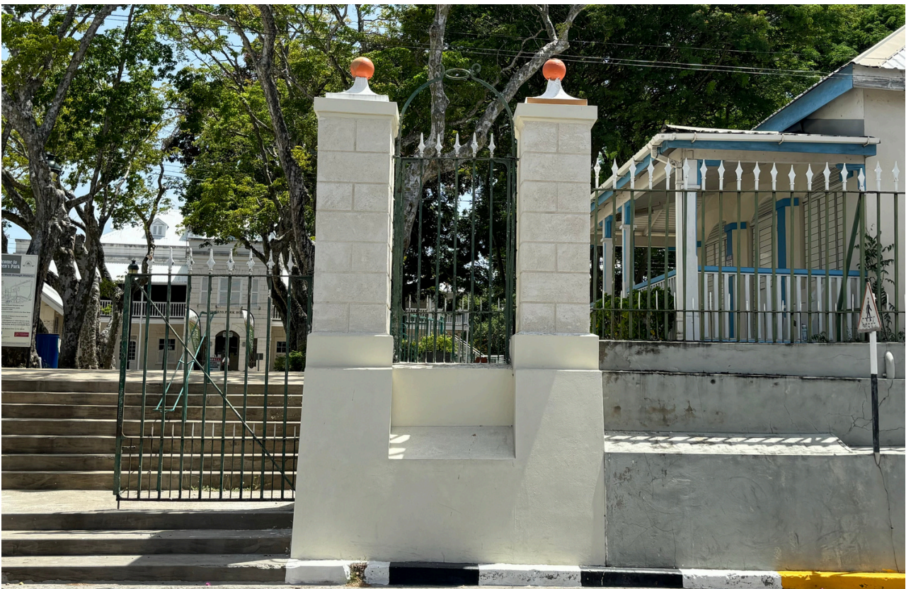
The other pair of the coral rendered gate columns after completion.
