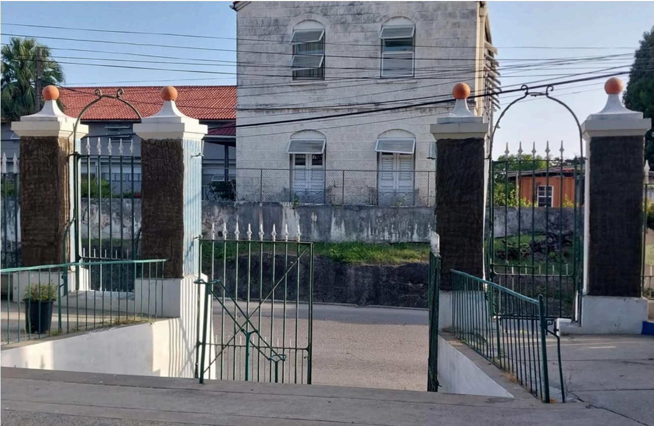
The columns' bases were painted after the completion of the coral rendering.
