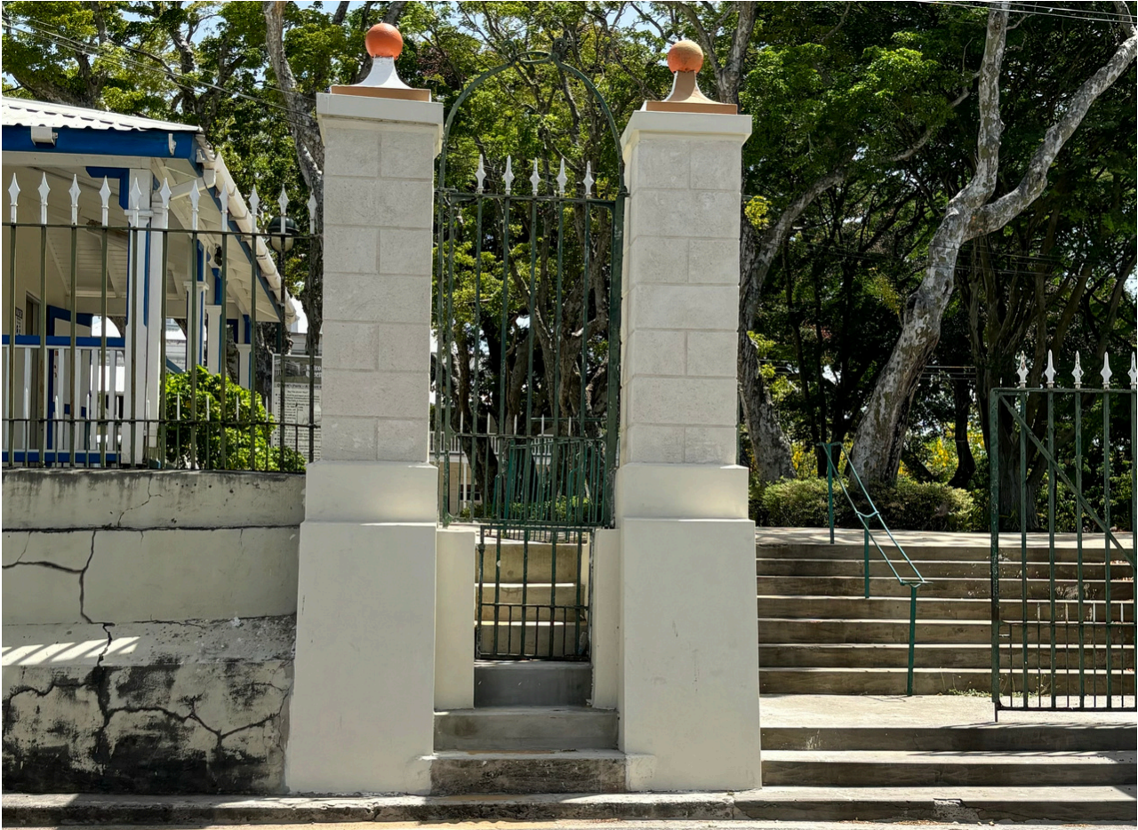
A pair of the coral rendered gate columns after this phase was completed.
