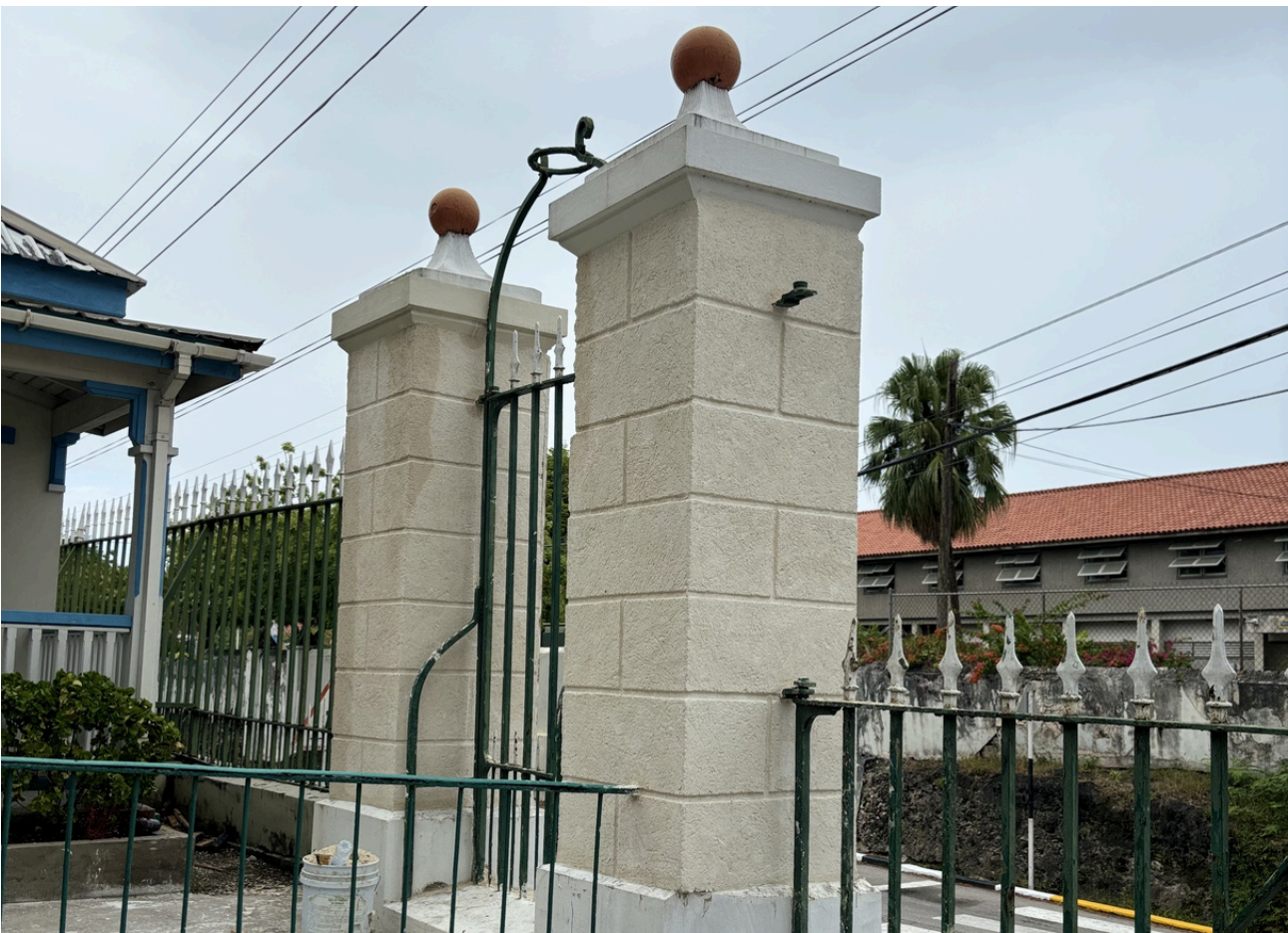
The coral rendered design of the columns before the water glaze was applied.
