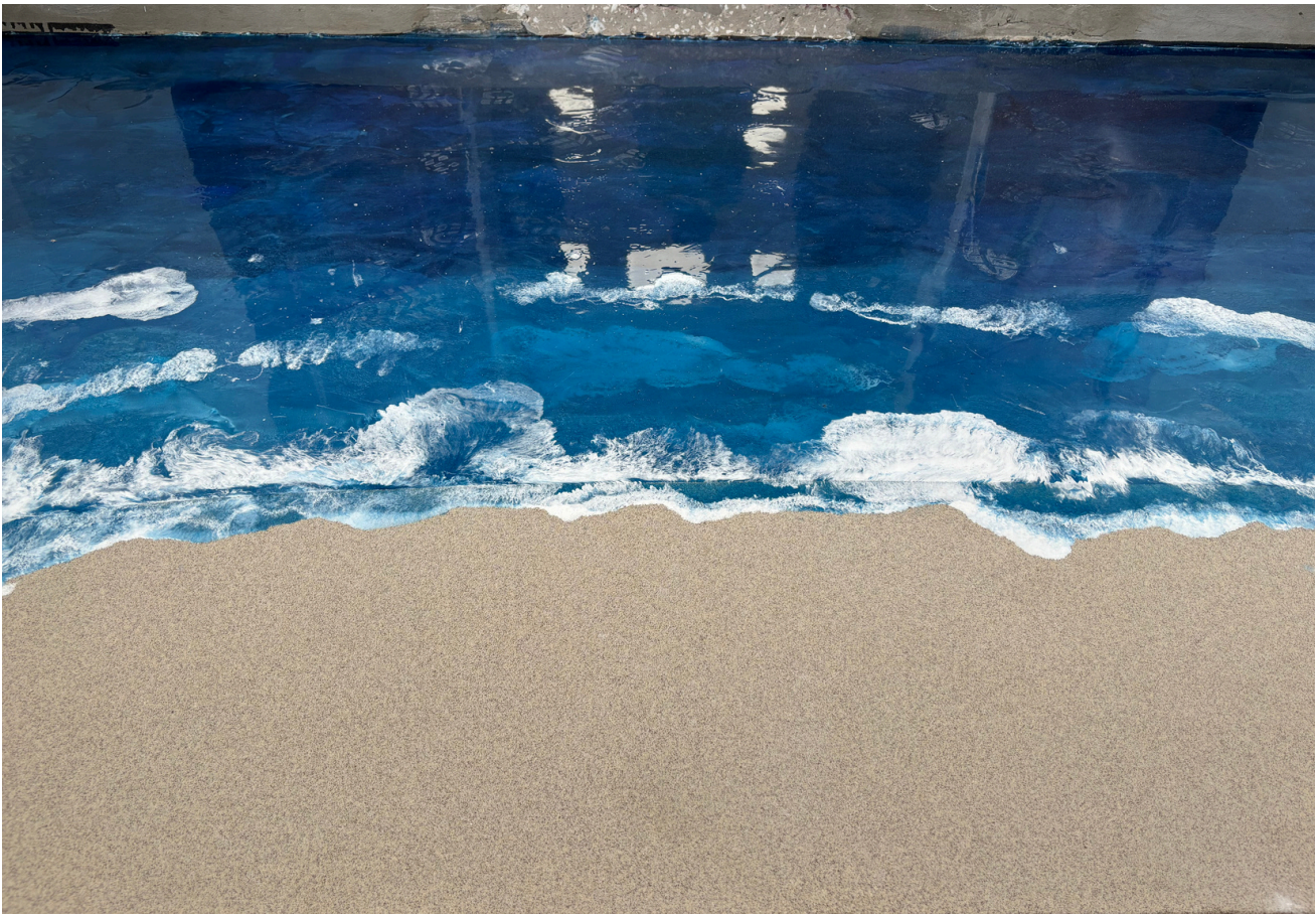
The beach-themed epoxy floor at Codrington House’s entryway is taking shape.
