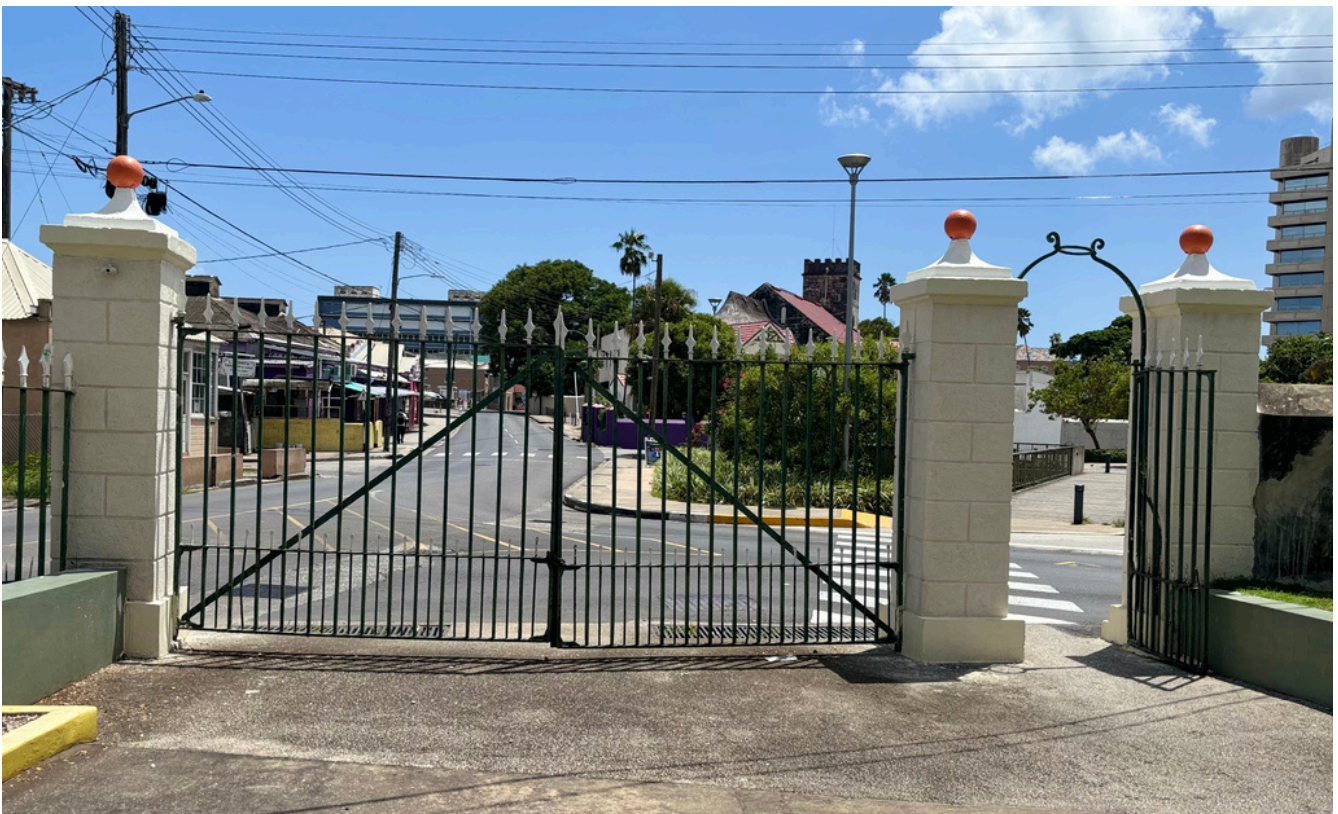
The coral rendering of Nelson’s Gate Columns was the final phase of this project.
