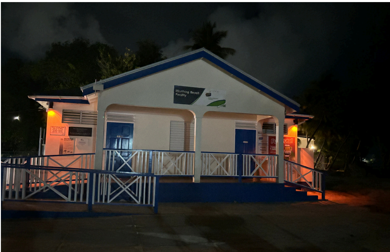
Four turtle-friendly lights were recently installed at the Worthing Beach Facility.
