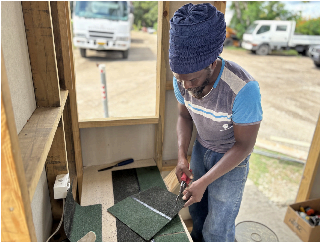
Artisan, Junior Sealy, cutting the materials for the shingles application on the roof.
